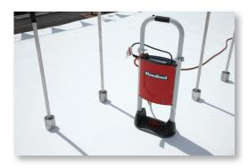
With the Firestone UltraPly TPO InvisiWeld system the wind load is distributed evenly across the roof, improving overall roof performance. With the traditional fastening method the load is concentrated at the seams. The UltraPly TPO InvisiWeld system achieves an FM 1-90 rating or above. In static testing, the InvisiWeld system bond resists over 500 lb<sub>f</sub> (2.2 kN) of force.
