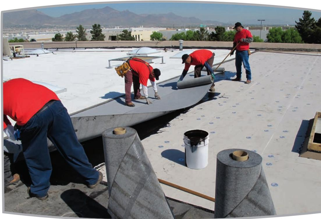
New LiquiGard Membrane Adhesive is economical, odorless and contains zero VOC, improving conditions for installers. The 2-part urethane adhesive forms extremely strong bonds between roofing membranes, insulation and substrates, creating superior resistance to high winds. LiquiGard adhesive is ideal for schools, hospitals and other applications where using hot asphalt, heat welding with torches or smelly solvents is not acceptable.
